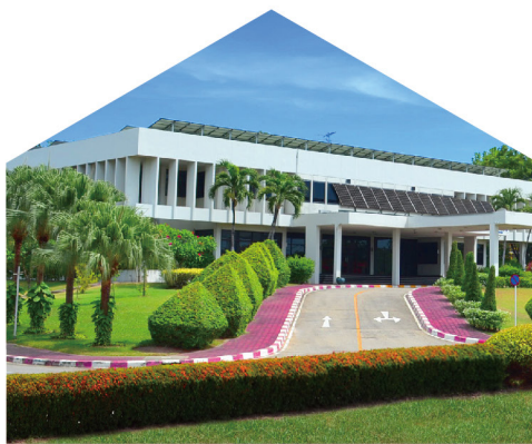
Siam Compressor Industry Co., Ltd
