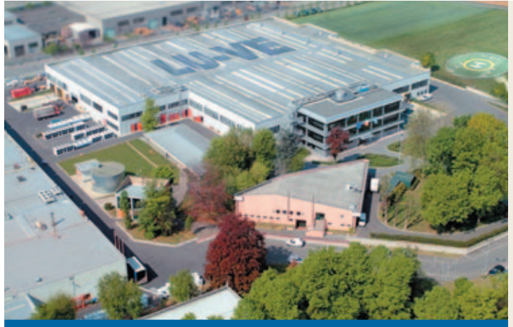
Partial view of the plant - UBOLDO
