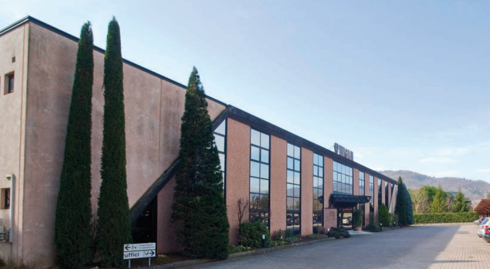
Castel San Niccolò (Italia) Headquarter
